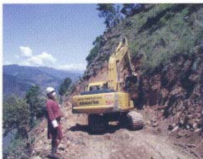
Road formation cutting and disposing surplus earth to safe place
