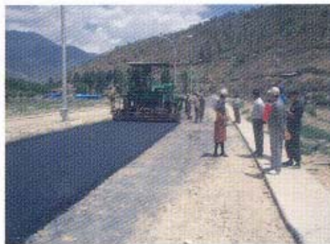
Mechanized road surfacing
