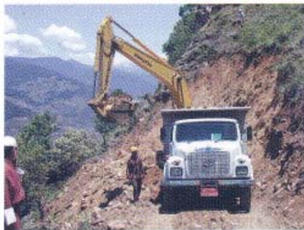
Road formation cutting and disposing surplus earth to safe place
